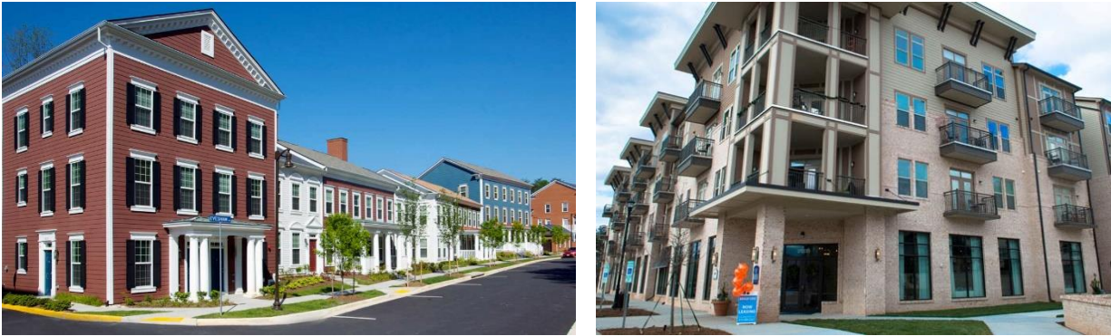
Figure 5.7.D(5)c: Examples of Front Façades
